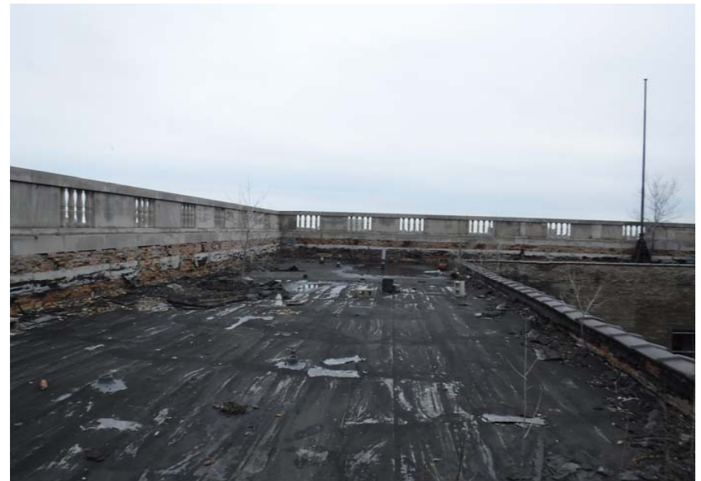
ROOF TOP V: Note ponding and deteriorated brickwork and limestone parapets.
