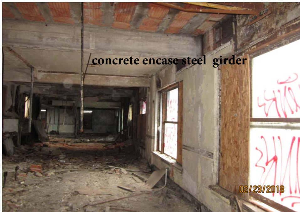
TYPICAL STRUCTURAL COMPOSITE CONCRETE CLAY-TILE FLOOR , Note concrete encased steel beams and columns . Underside of floors in good condition. View at the underside of 3r, 4th floors and roof. Page 3
