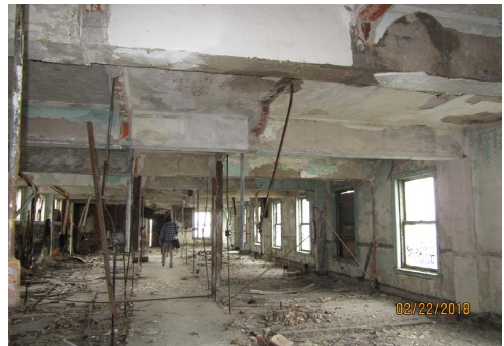
TYPICAL STRUCTURAL COMPOSITE CONCRETE CLAY-TILE FLOOR , Note concrete encased steel beams and columns . Underside of floors in good condition. View at the underside of 3r, 4th floors and roof. Page 3
