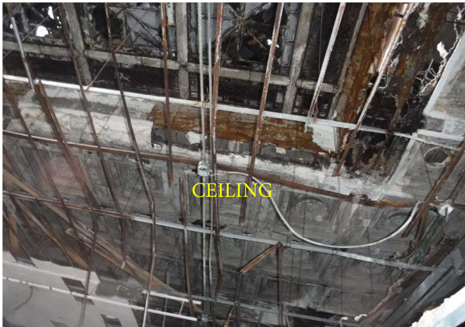
VIEWS OF THE MAIN ATRIUM FLOOR ( 2nd Floor), Note loose ceiling tiels, framing, and finishings. Page 5
