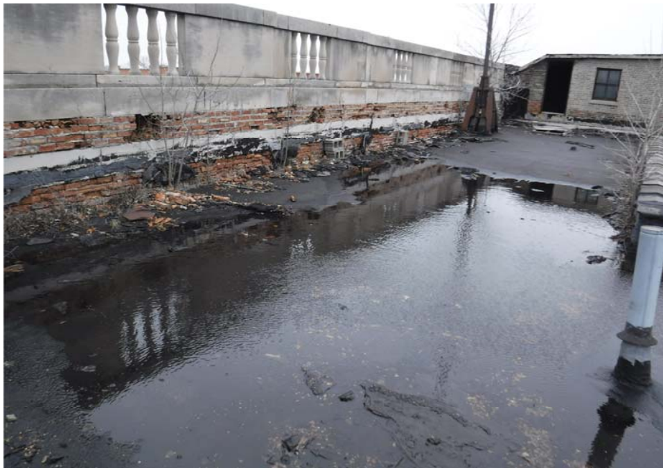
ROOF TOP V: Note ponding and deteriorated brickwork and limestone parapets.
