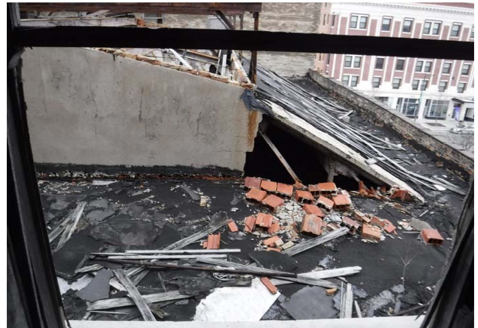
ATRIUM CEILING FRAMING SUPPORTED BY 3rd FLOOR. Note loose secondary framing of atrium roof which not a part of main structural framing of the building. Main steel framing was not visible.
