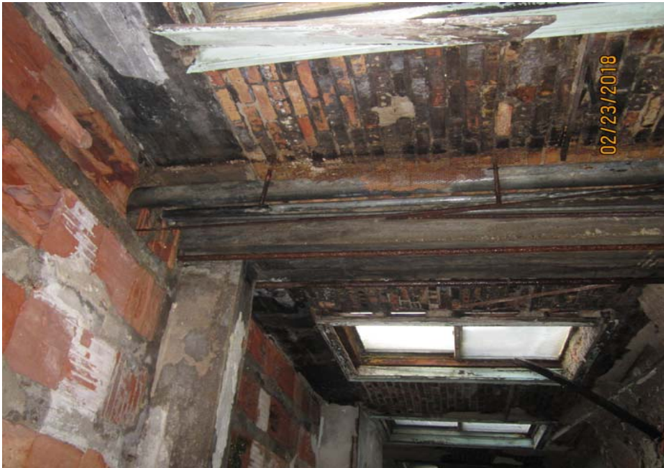
TYPICAL CONSTRUCTION DETAILS : Note interior facing of perimeter masonry walls, steel stairs, and perimeter concrete encased steel columns found to be in sound condition.
