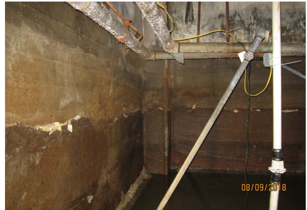
BASEMENT PERIMETER WALLS AND CONCRETE ENCASED INTERIOR COLUMNS . NOTE GOOD CONDITION OF WALLS AND COLUMNS.
