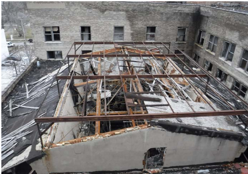
ATRIUM CEILING FRAMING SUPPORTED BY 3rd FLOOR. Note loose secondary framing of atrium roof which not a part of main structural framing of the building. Main steel framing was not visible.
