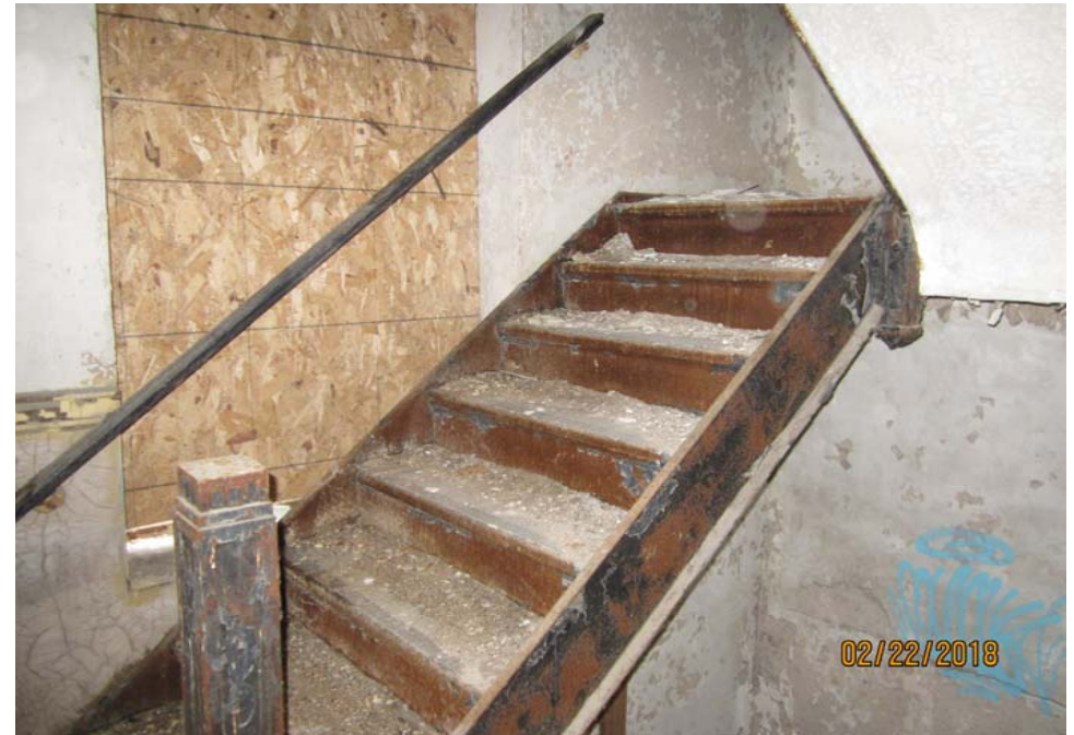
TYPICAL CONSTRUCTION DETAILS : Note interior facing of perimeter masonry walls, steel stairs, and perimeter concrete encased steel columns found to be in sound condition.
